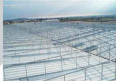
The main element that composes this product is the **Truss**, which is a beam of shaped lattice made of tubular and rectangular shapes and assembled by screws or weld, the execution of this work is executed always in workshop, and under the most demanding measures of control, the set is supplied the place of the installation with **the hot-dip galvanized surface treated**.
